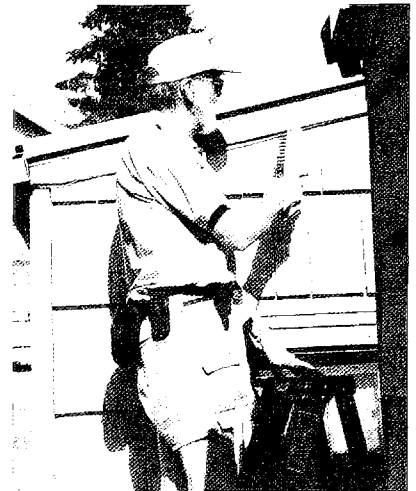
Dwight Williamson, DO, retired family planning, scrapes loose paint in preparation for primer and new paint
